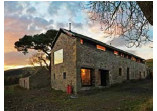
The Mill, Southside Steading
