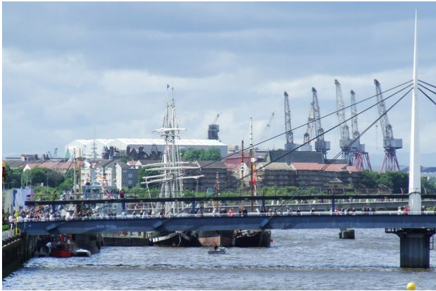
Cable stayed footbridge joining Dumfries and Lincluden
